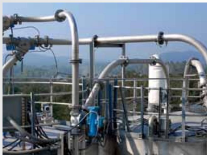
Dilute Phase Conveying System with Long Radius Elbows
